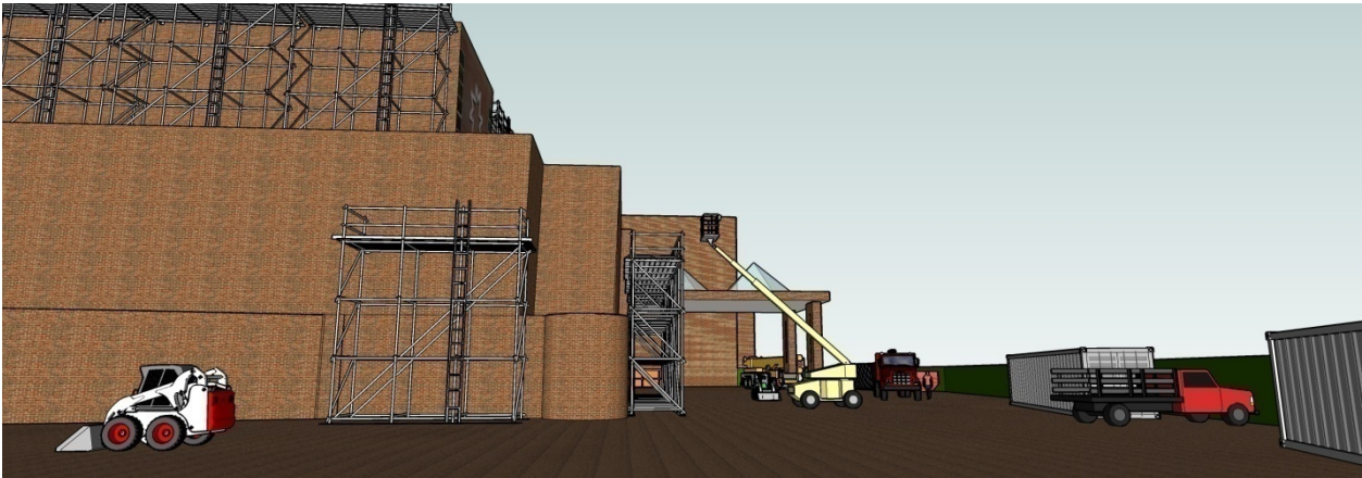
Figure 5 – View of Southeast corner
